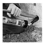
Slightly raise the cable/pipe and apply STOPAQ® with the sealant gun. Inject at least 100 mm of the sealing compound into the recess.
