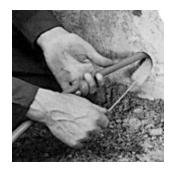
Thoroughly clean the recess with a brush, following up with a water jet if necessary. STOPAQ® will even stick to a wet substrate. The temperature of the substrate must not be higher than 50°C.
