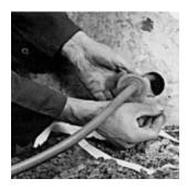
Wind foam tape around the cable/pipe but do not stick it to it, i.e. do not remove the protective backing strip from the adhesive coat of the first winding. The diameter of the tape must be 1 cm (1-2 windings) greater than the diameter of recesses. Wind the tape tightly.
