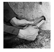
Push the tape into the recess with a spatula. The distance from the start of the recess to the tape should be at least 100 mm. Make sure that the tape seals off the recess effectively.
