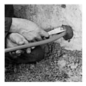
Finally, apply and press STOPAQ® around the cable and recess with a spatula. The use of STOPAQ® mortar is recommended to make cable/pipe glands pressure-tight to 0.5 bar.
