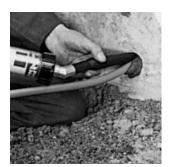
When the recess is properly filled, some improvements can be carried out where necessary. Push the cable downwards until it rests against the recess and, if necessary, apply more sealing compound.
